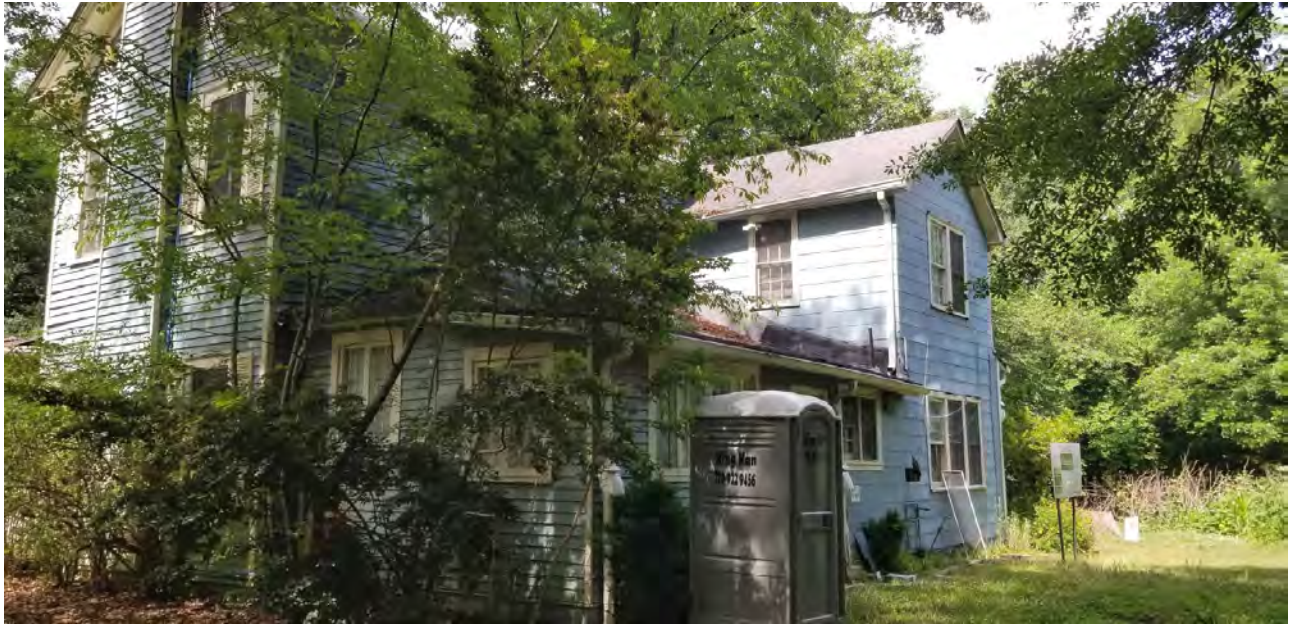
PHOTO 50: (View of South West Façade, at rear corner):
