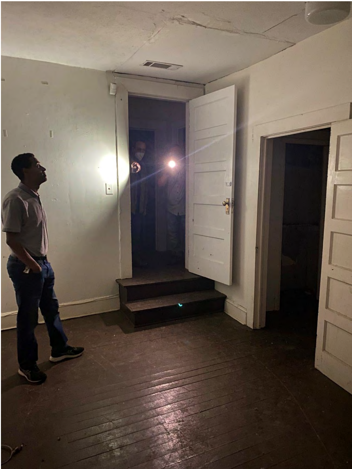
PHOTO 124: (View of Interior, Room 8, 2 nd Floor)
