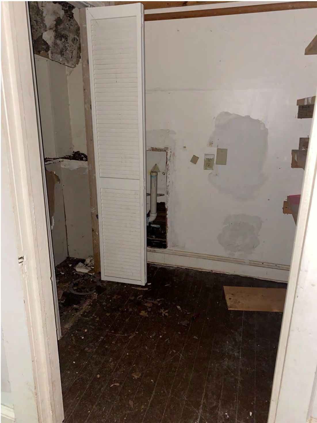
PHOTO 129: (View of Interior, Room 8, 2 nd Floor, large closet at front of room)
