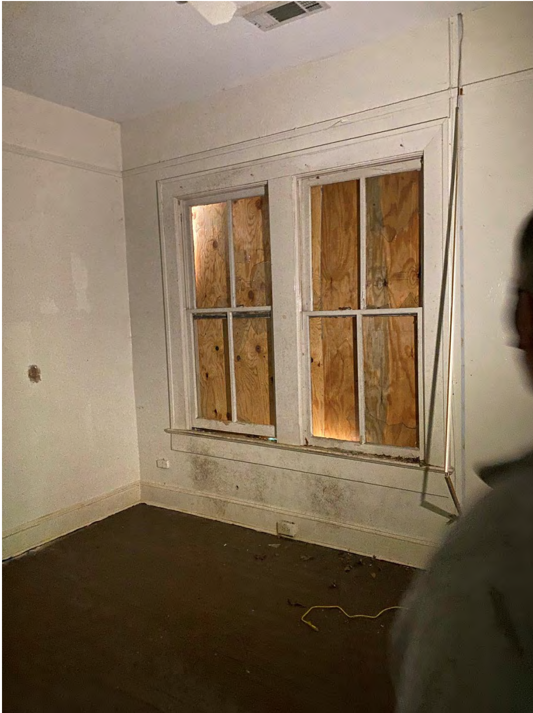
PHOTO 111: (View of Interior, Room 6, 2 nd Floor)
