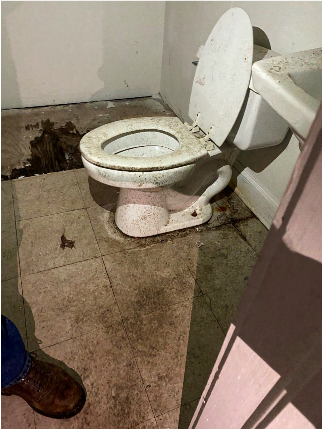
PHOTO 135: (View of Interior, bathroom, 2 nd Floor)
