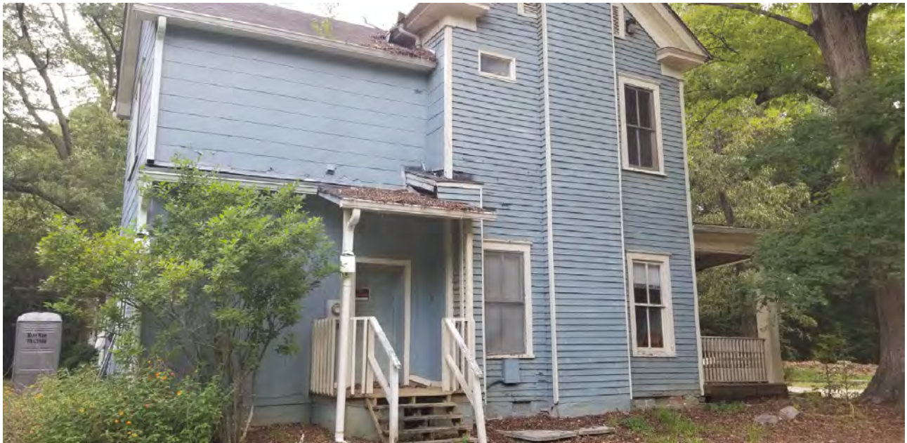
PHOTO 47: (View of East Façade):
