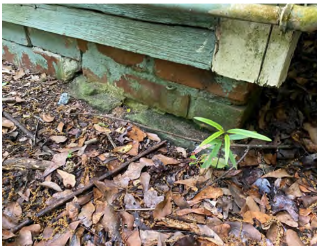
PHOTO 34, & 35: (View of Rear Façade, at South West corner):
