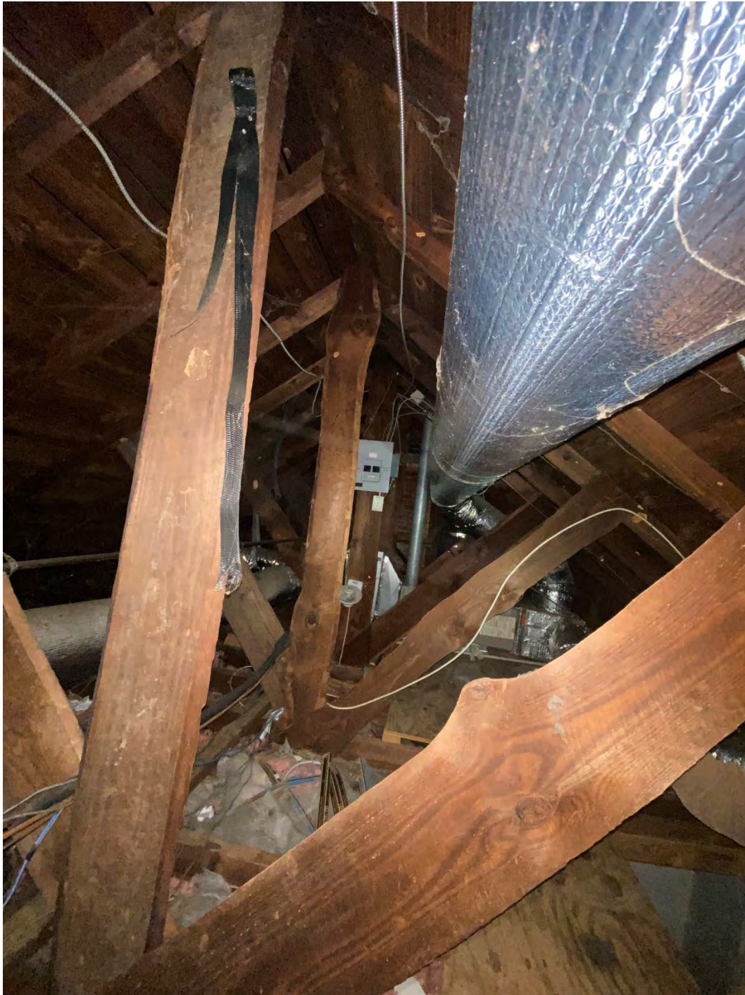
PHOTO 101: (View of Interior, attic, above main stairs)
