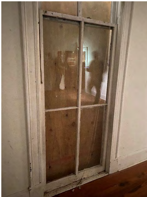
PHOTO 89, 90, & 91: (View of Interior, Room 4)
