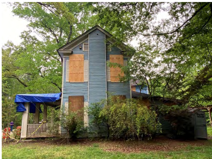
PHOTO 36: (View of West Facade):
