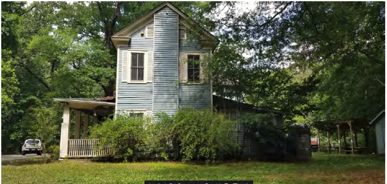
PHOTO 51: (View of West Façade at Main Structure):
