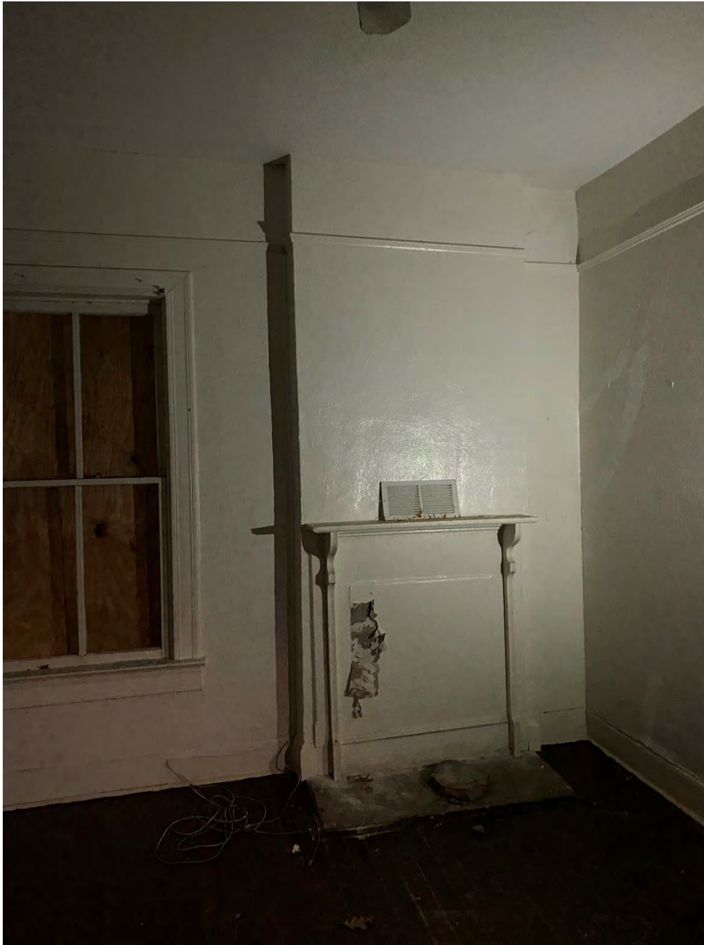
PHOTO 107: (View of Interior, Room 5, 2 nd Floor)
