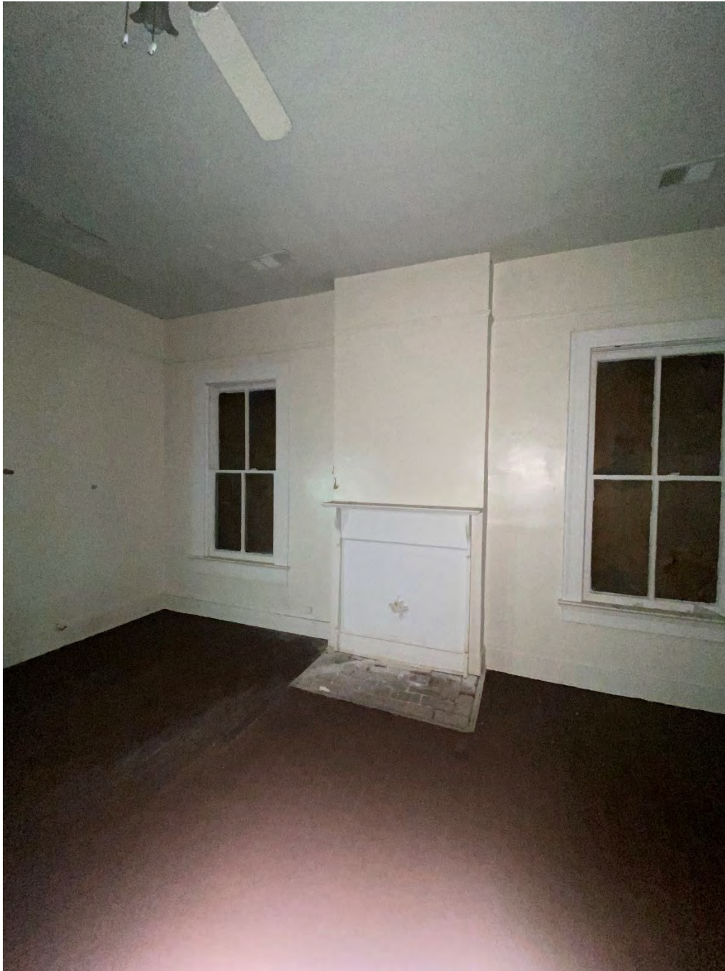
PHOTO 117: (View of Interior, Room 7, 2 nd Floor)
