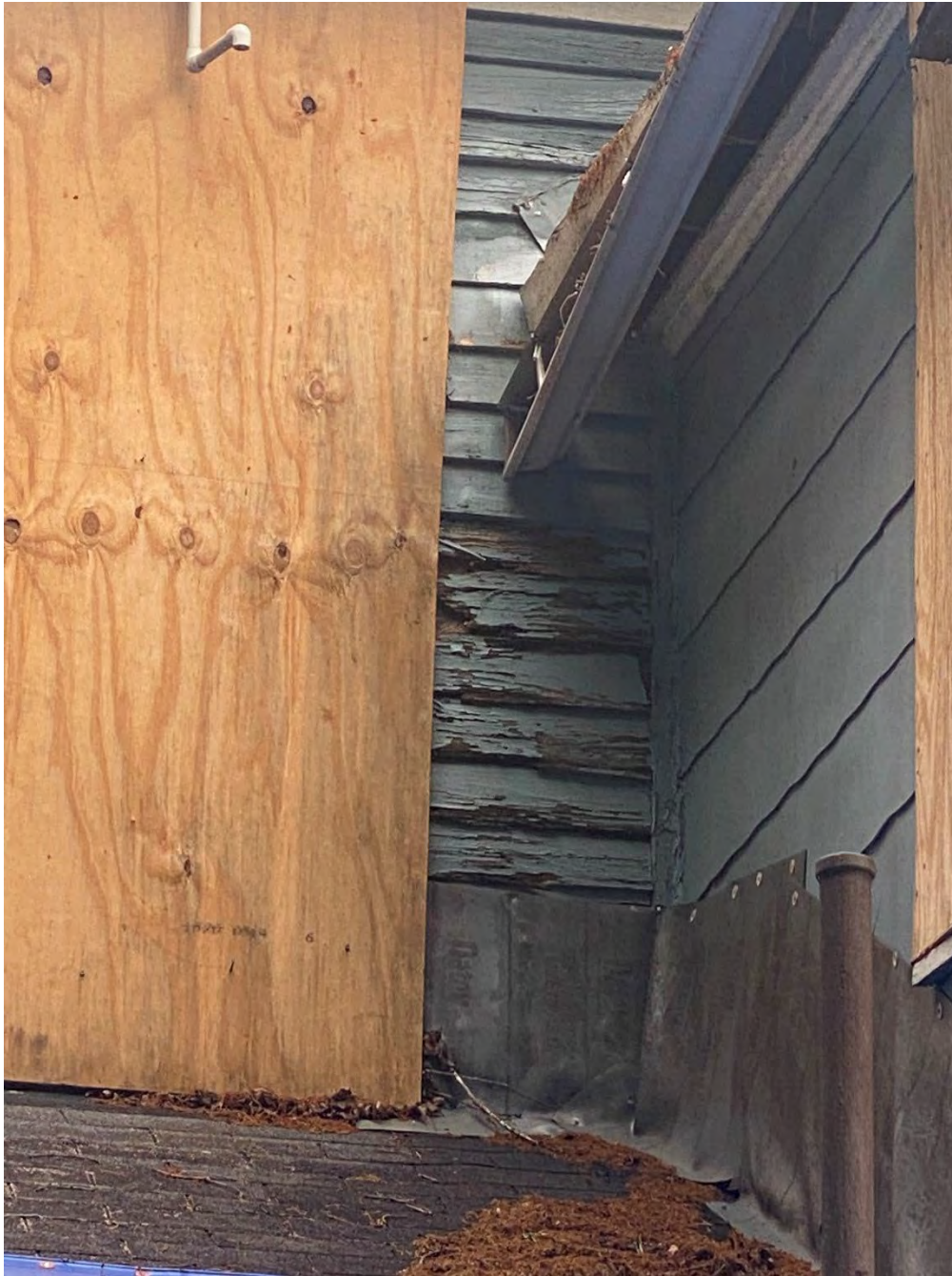
PHOTO 29: (View of Rear Facade): Main Structure transition to Addition 1,
