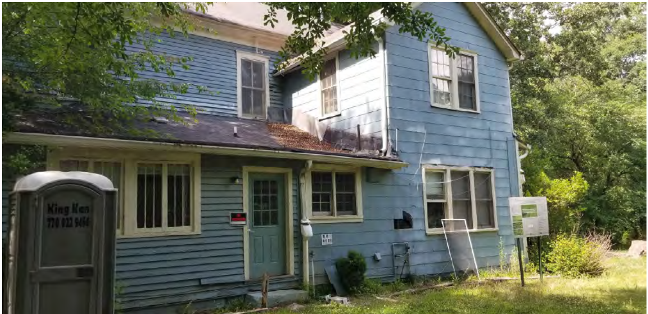
PHOTO 49: (View of South Façade, at rear):
