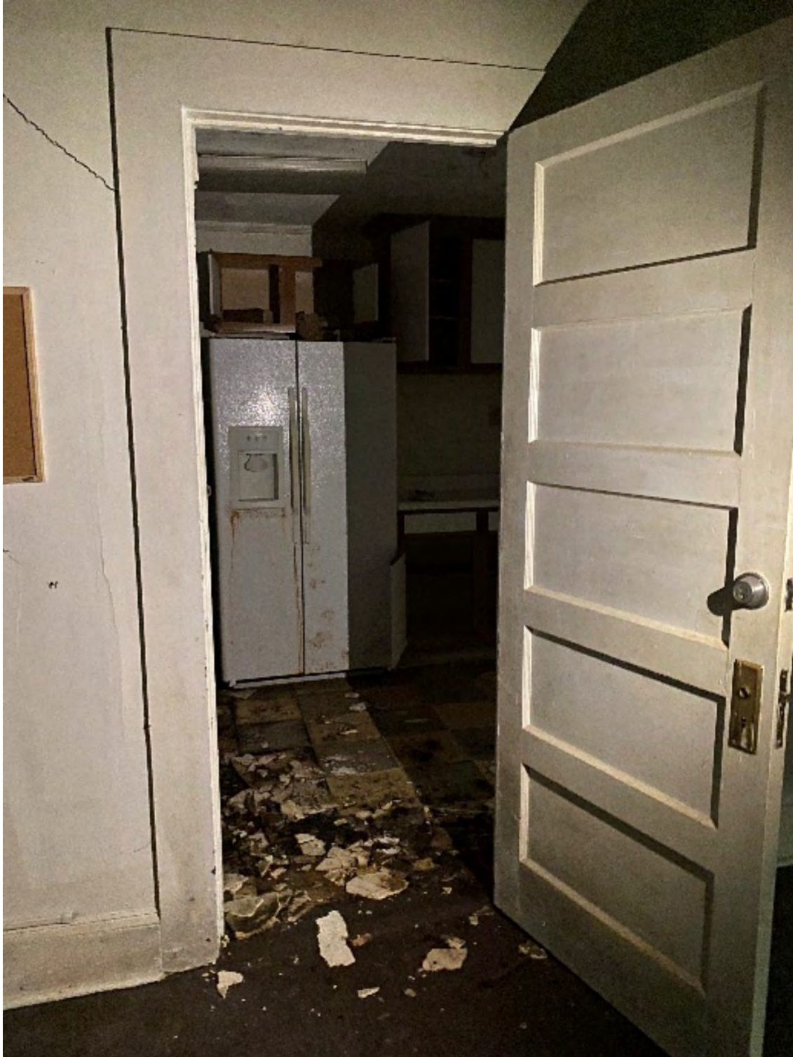
PHOTO 68: (View of Interior, Room 2, Addition 1, door to kitchen):
