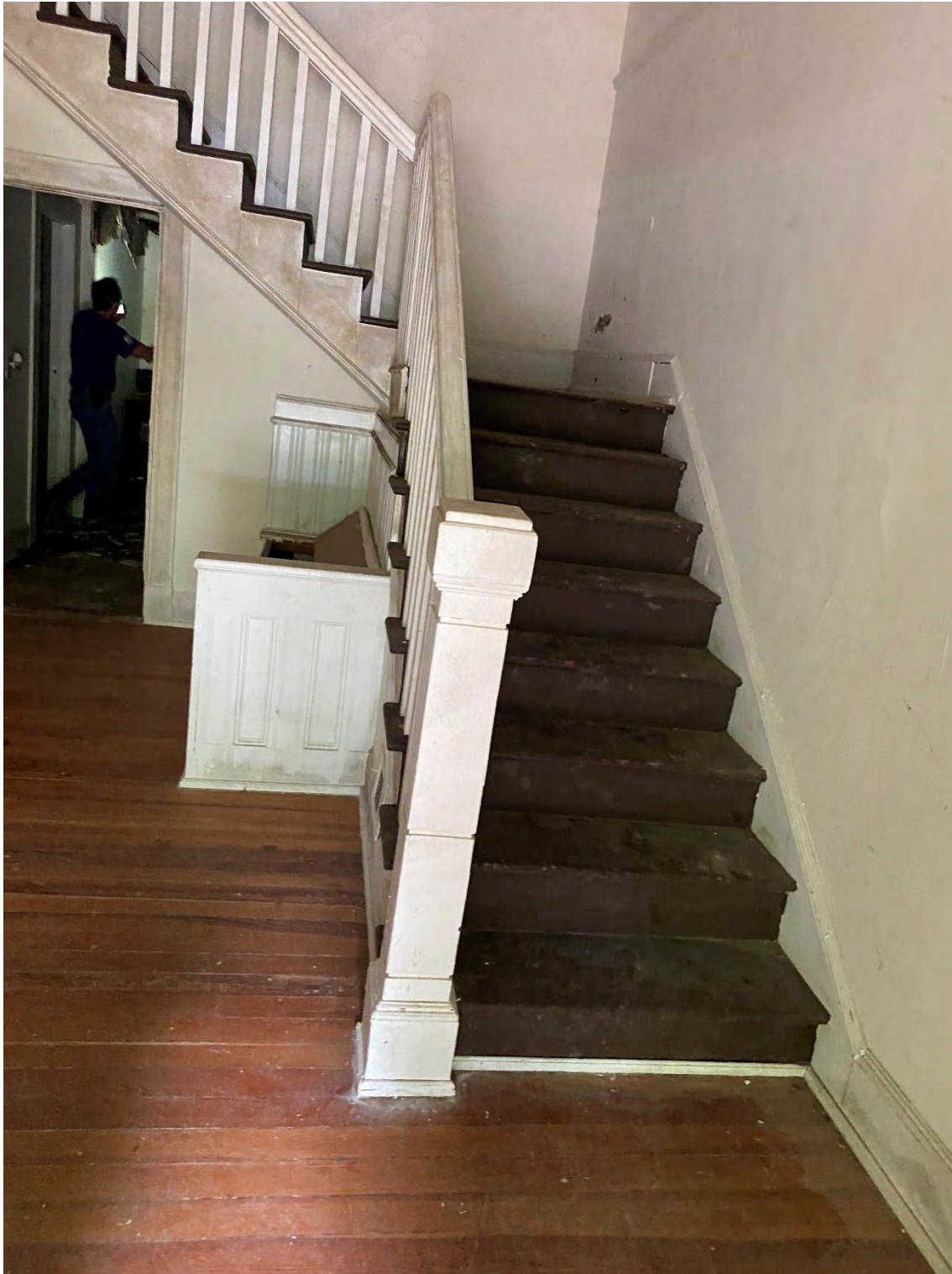
PHOTO 54: (View of Front, Interior at Foyer, at Main Structure):
