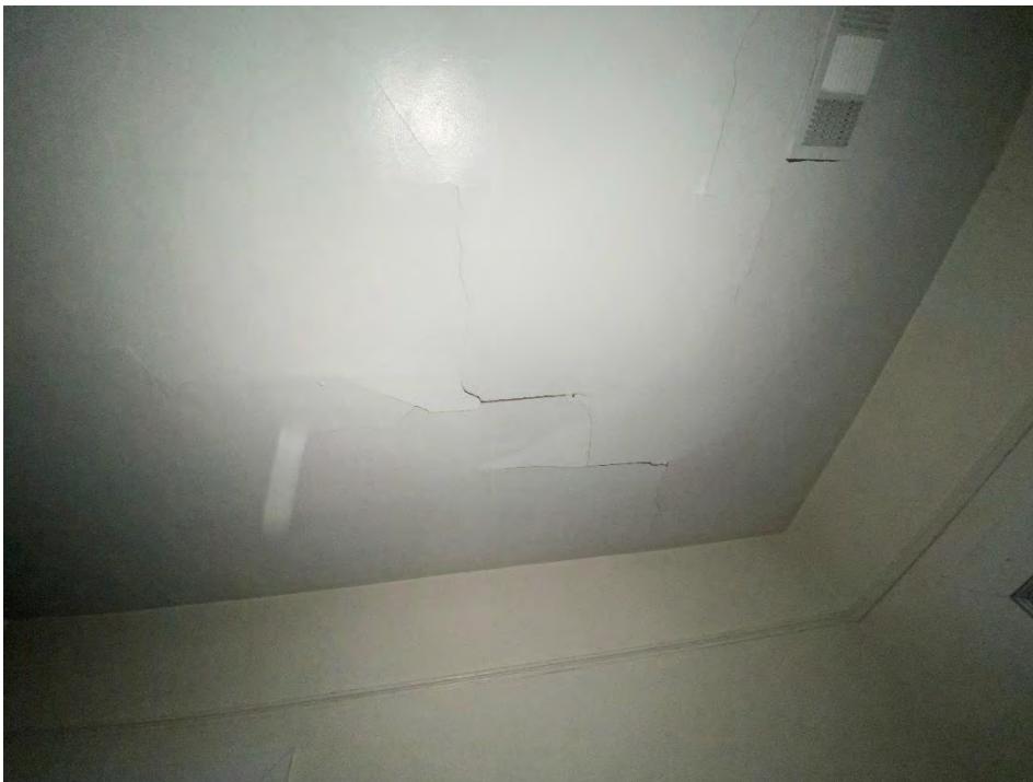
PHOTO 122: (View of Interior, Room 7, 2 nd Floor, ceiling)
