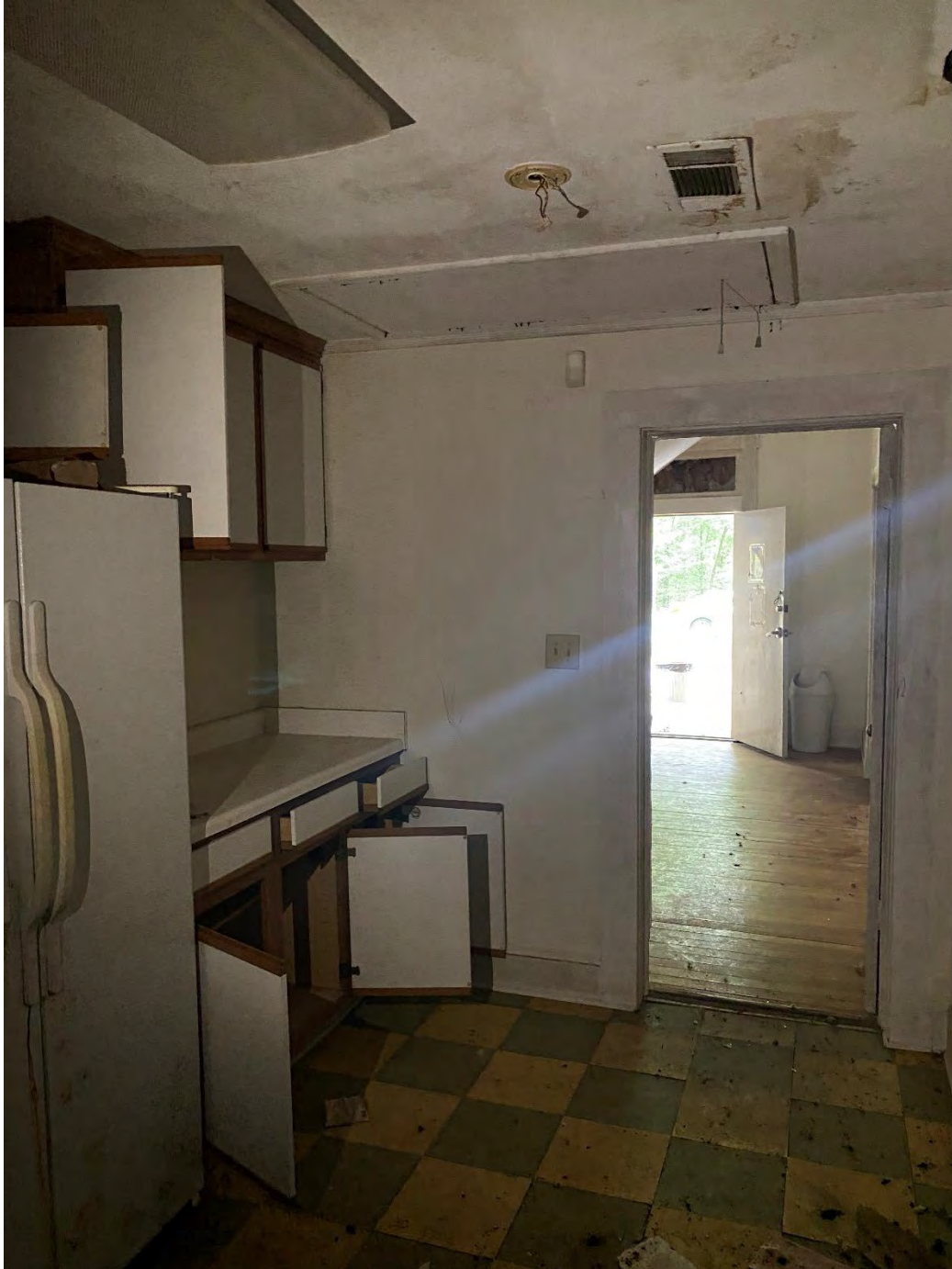
PHOTO 76: (View of Interior, Kitchen, Addition 1 & 2, view toward front entry):
