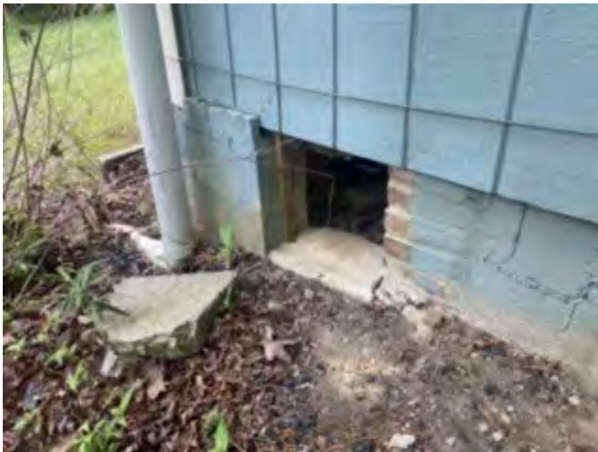
PHOTO 17: (View of East Façade Foundation – close up on T1-11 siding:
