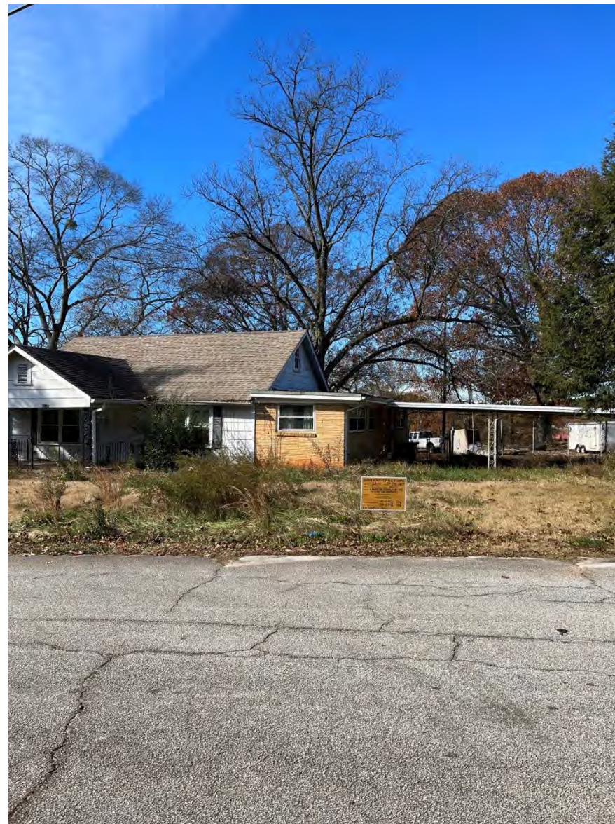
616 Woodland Avenue Scottdale, GA 30079 – Structure 1 of 2
