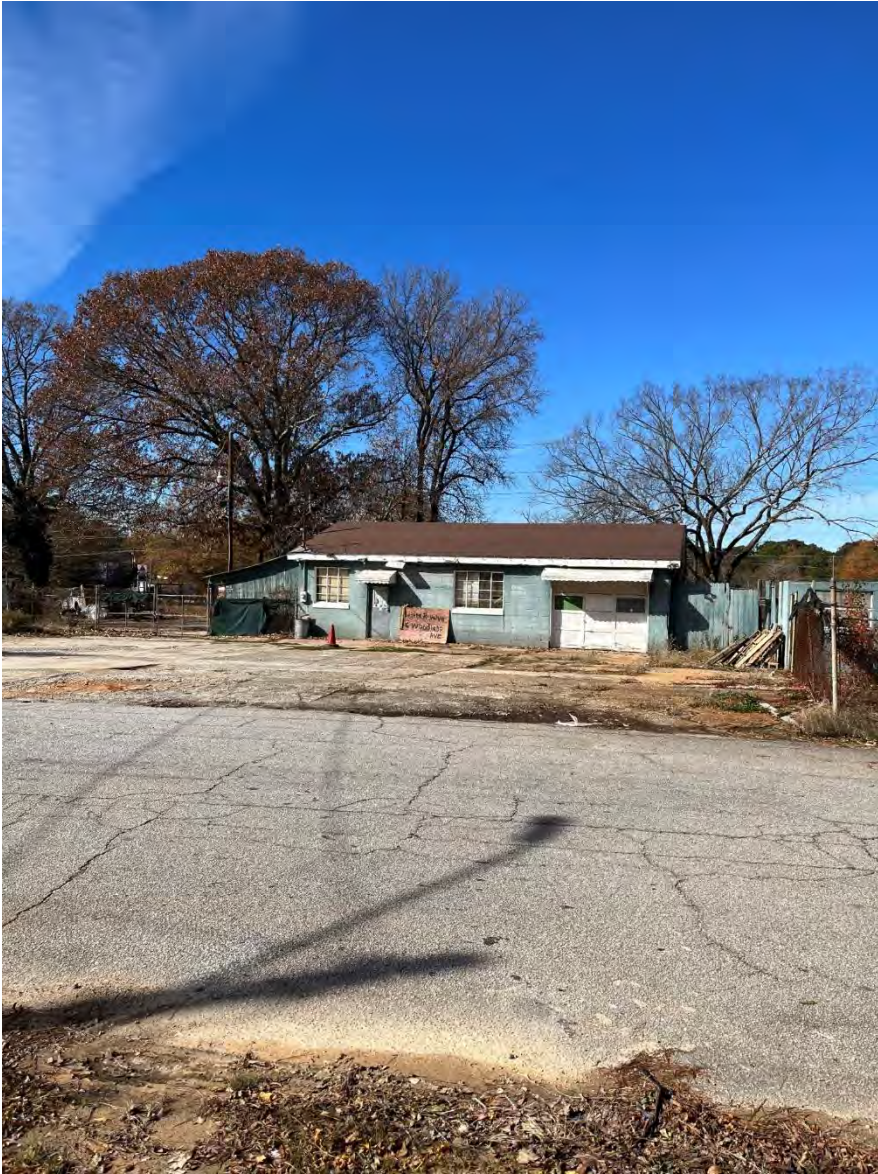
616 Woodland Avenue Scottdale, GA 30079 – Structure 2 of 2
