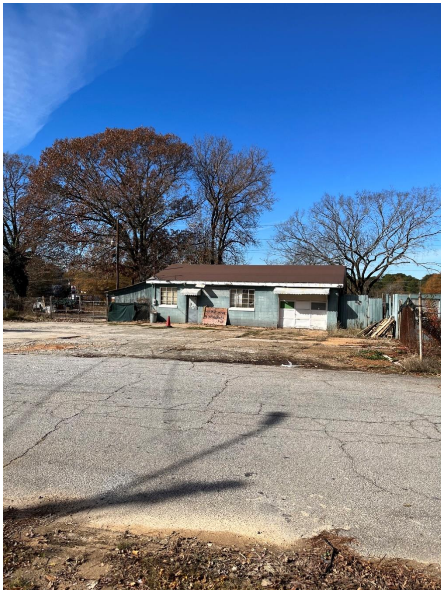
616 Woodland Avenue Scottdale, GA 30079 – Structure 2 of 2
