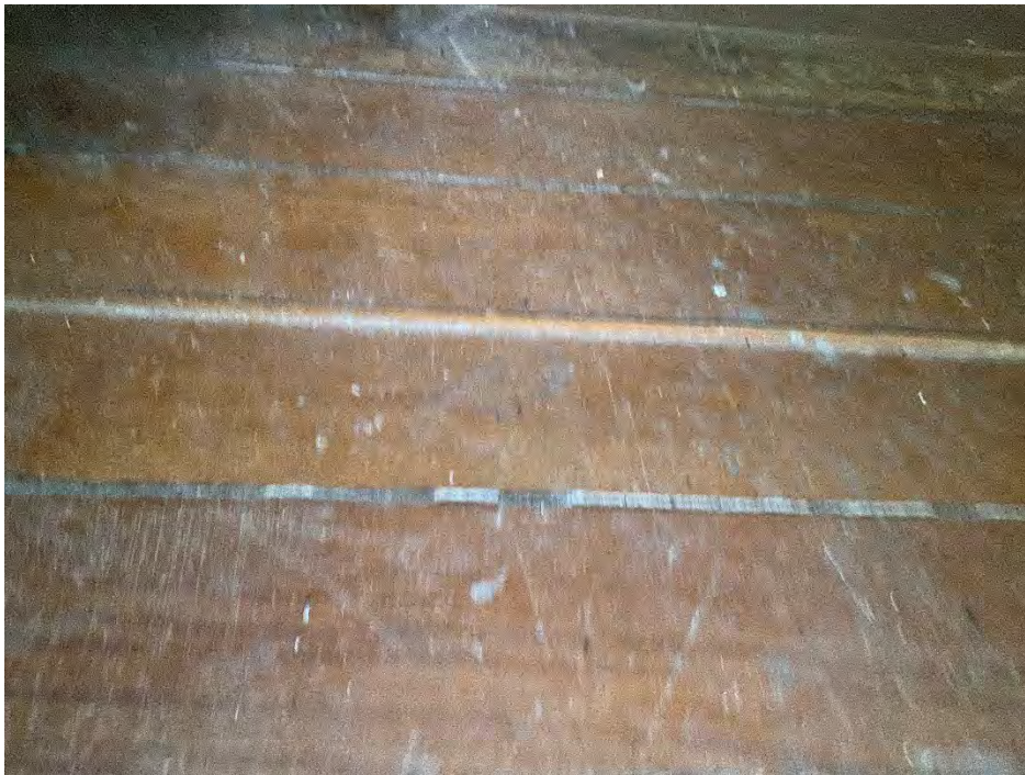
PHOTO 55 & 56: (View of Front, Interior at Foyer, at Main Structure, floor):
