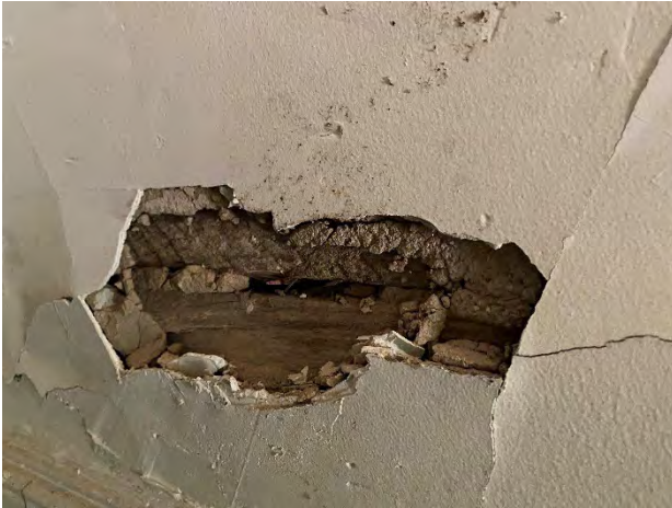
PHOTO 77, 78, & 79 : (View of Interior, Kitchen)
