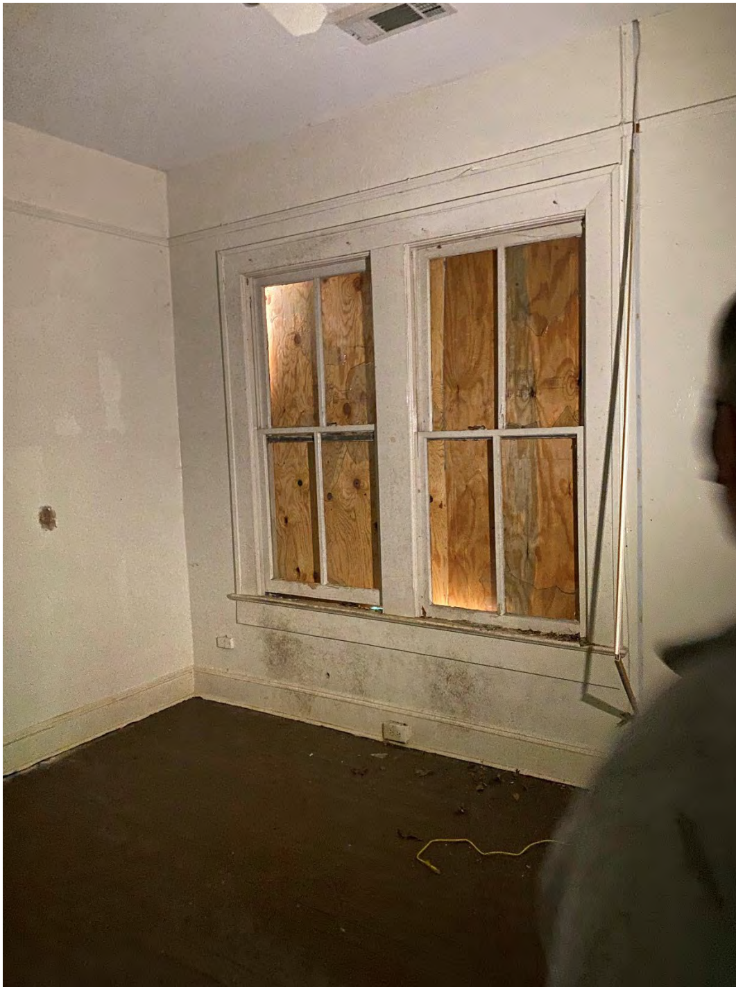
PHOTO 111: (View of Interior, Room 6, 2 nd Floor)
