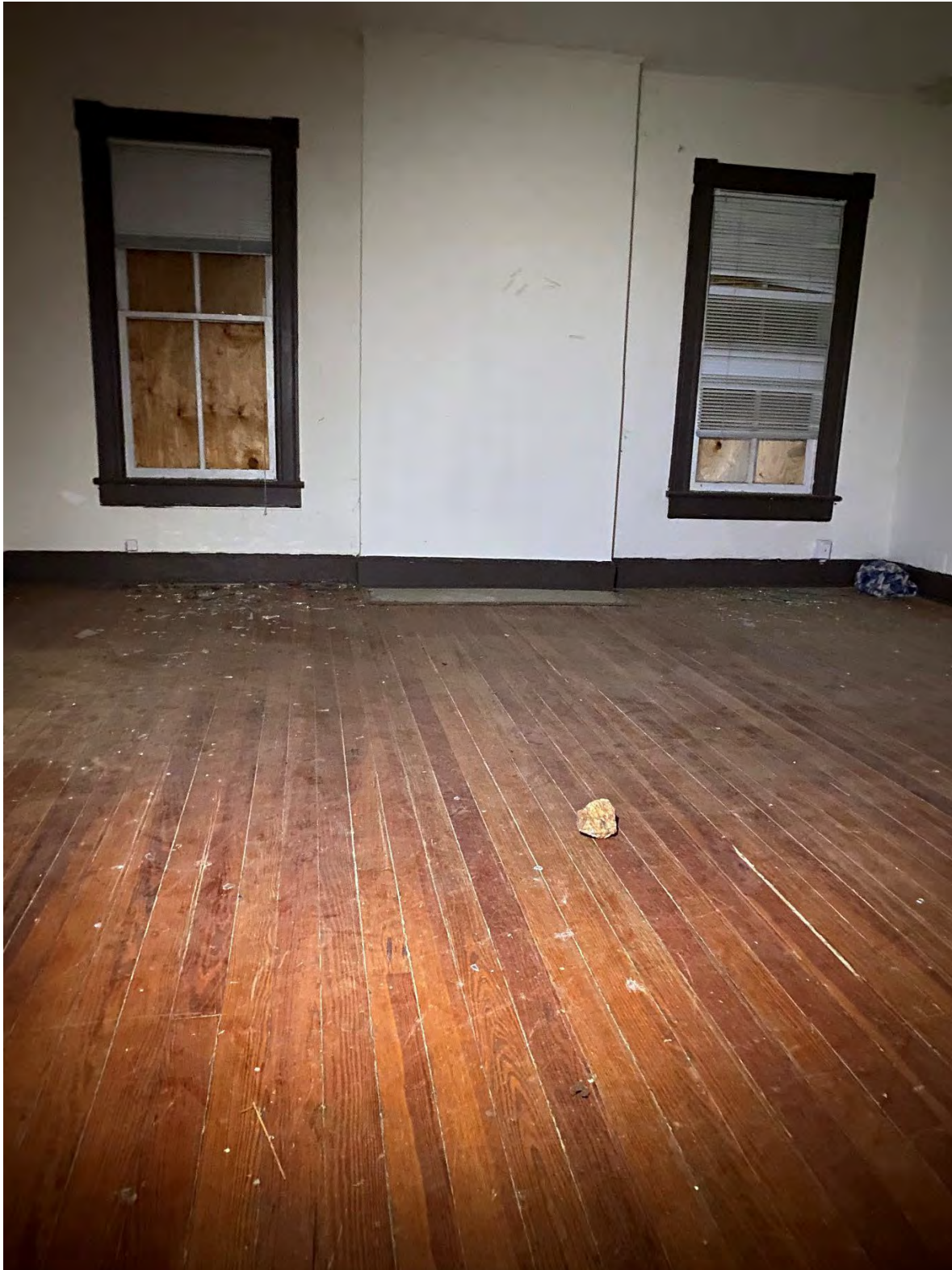
PHOTO 58: (View of Interior, Room 1):
