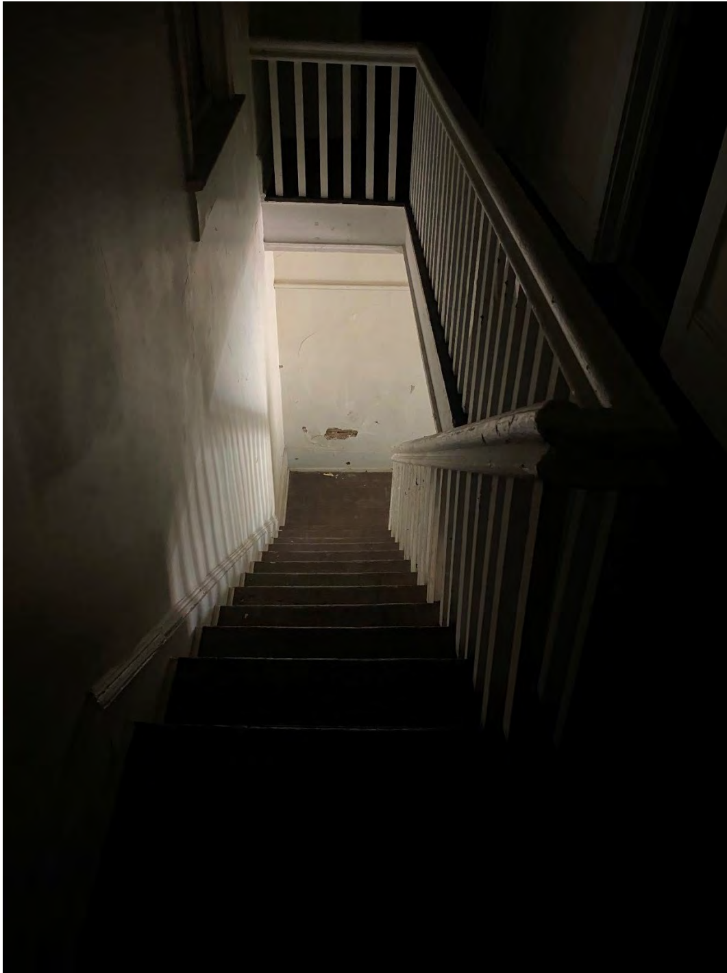
PHOTO 141: (View at 2 nd Floor, at top of stair, looking downward)
