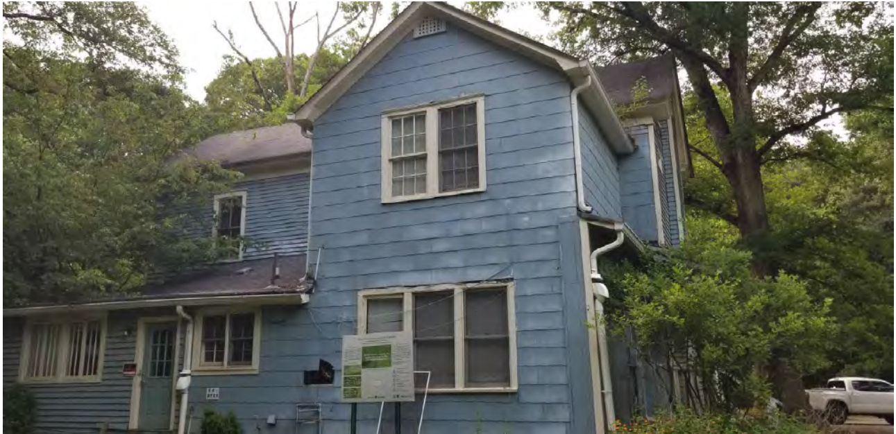
PHOTO 48: (View of South Façade, at rear):
