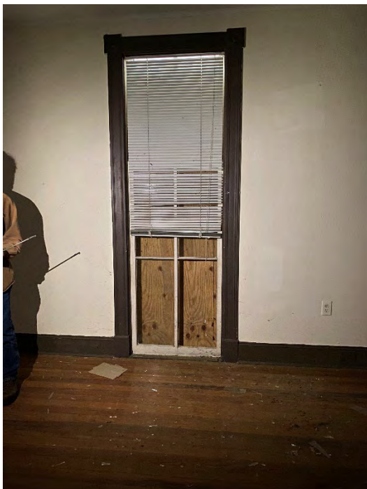
PHOTO 60 & 61: (View of Room 1, Ceiling, and Window)
