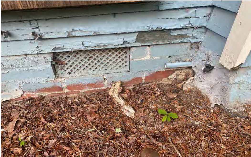
PHOTO 16: (View of East Façade Foundation – close up on brick infill & venting):
