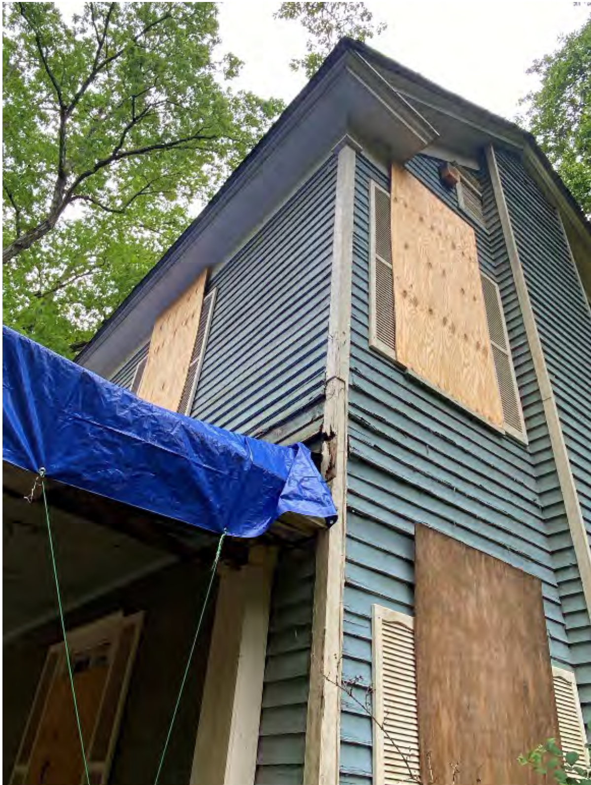
PHOTO 40: (View of West Façade at Main Structure, at Porch connection, close-up).
