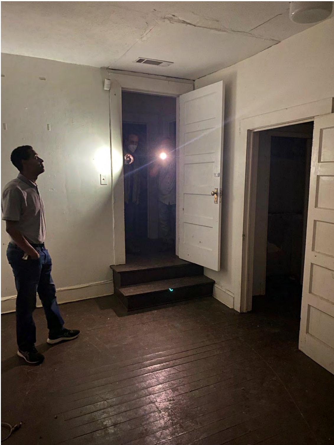
PHOTO 124: (View of Interior, Room 8, 2 nd Floor)
