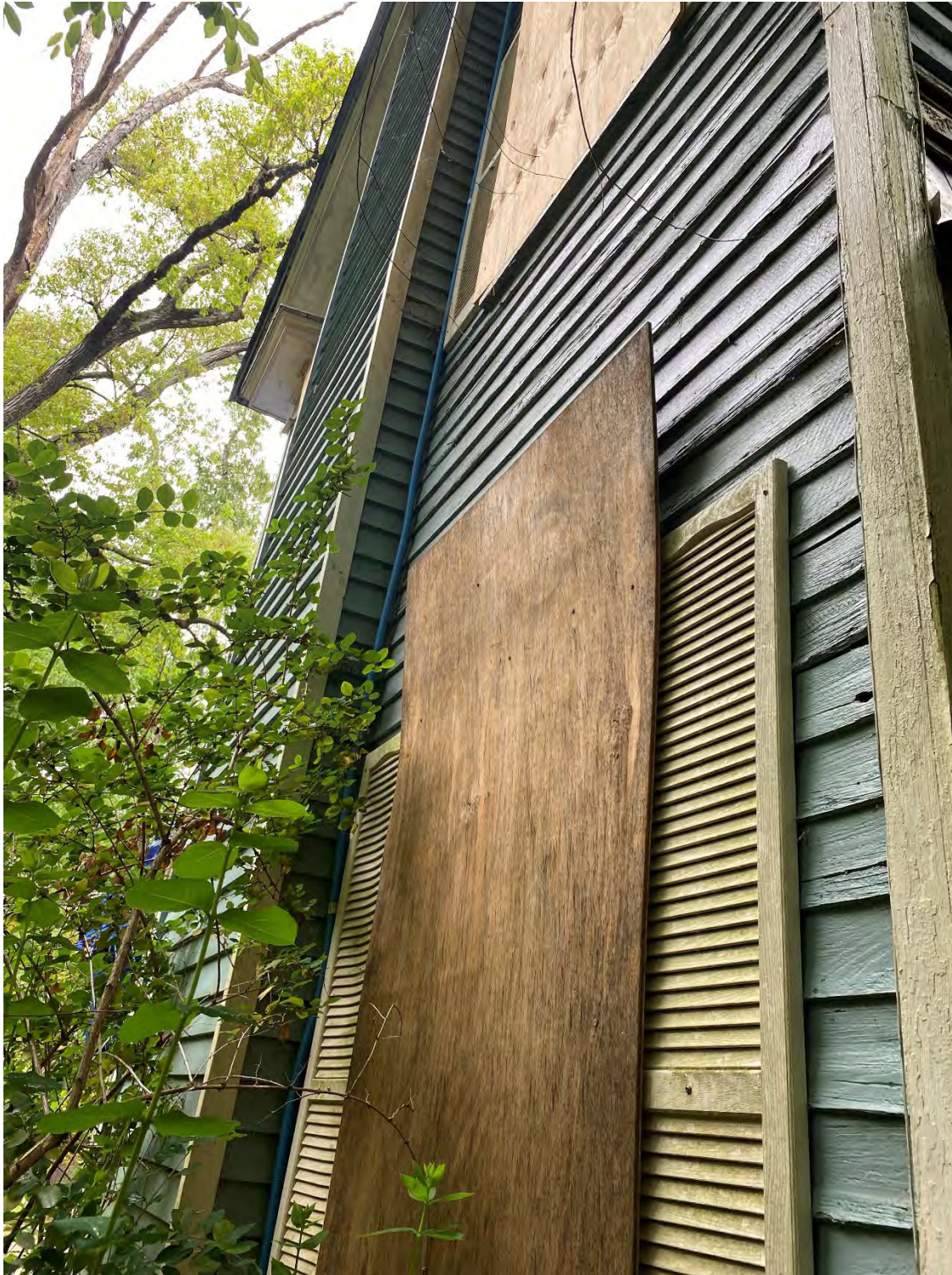
PHOTO 37: (View of West Façade at Main Structure, close-up):
