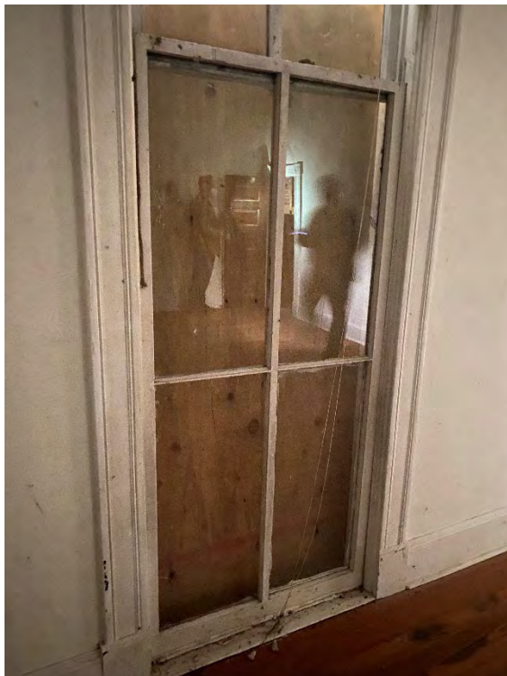
PHOTO 89, 90, & 91: (View of Interior, Room 4)
