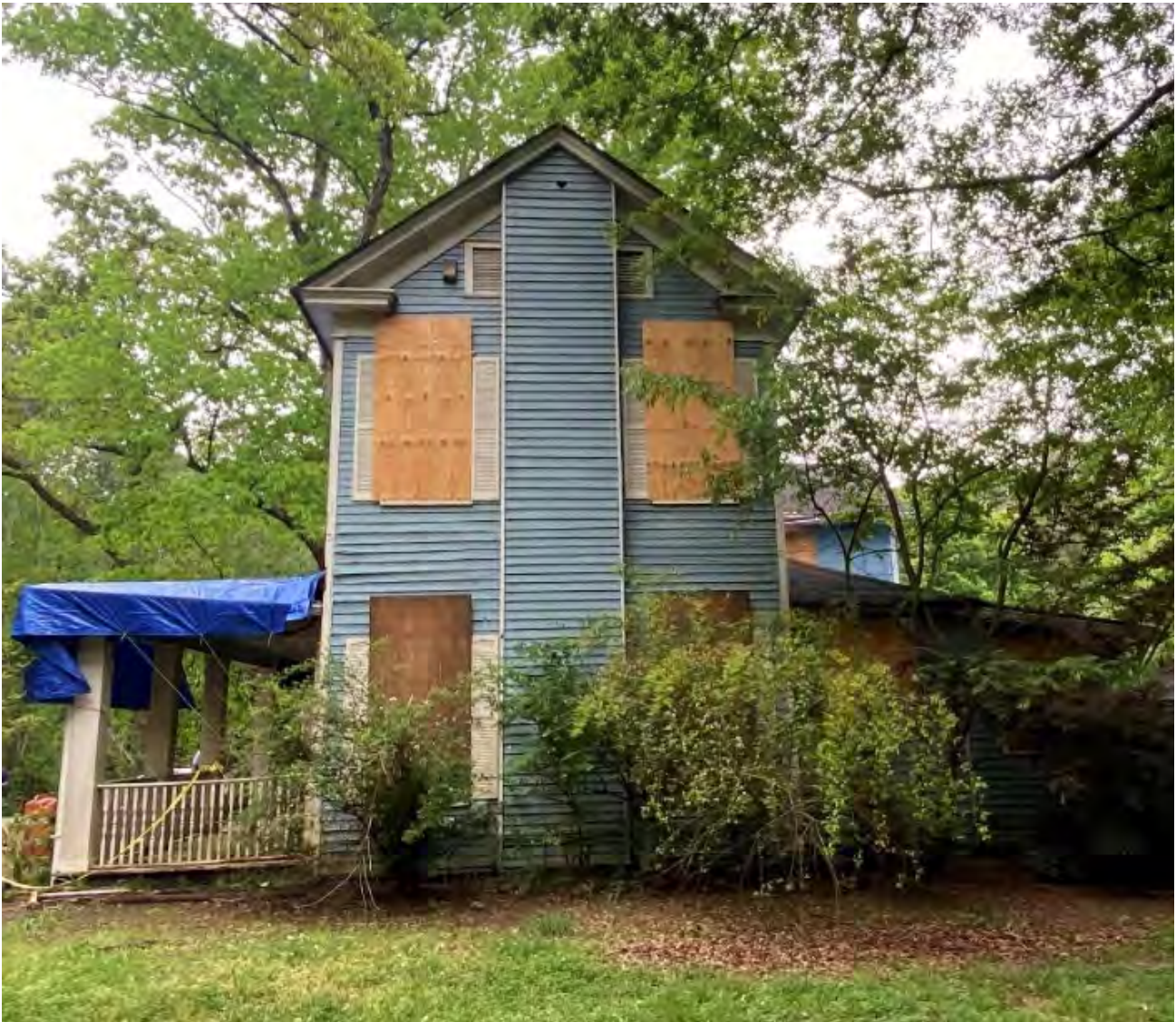
PHOTO 36: ENLARGED (View of West Facade):
