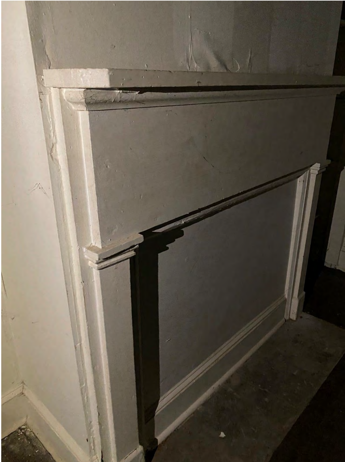
PHOTO 64: (View of Interior, Room 2, Addition 1):
