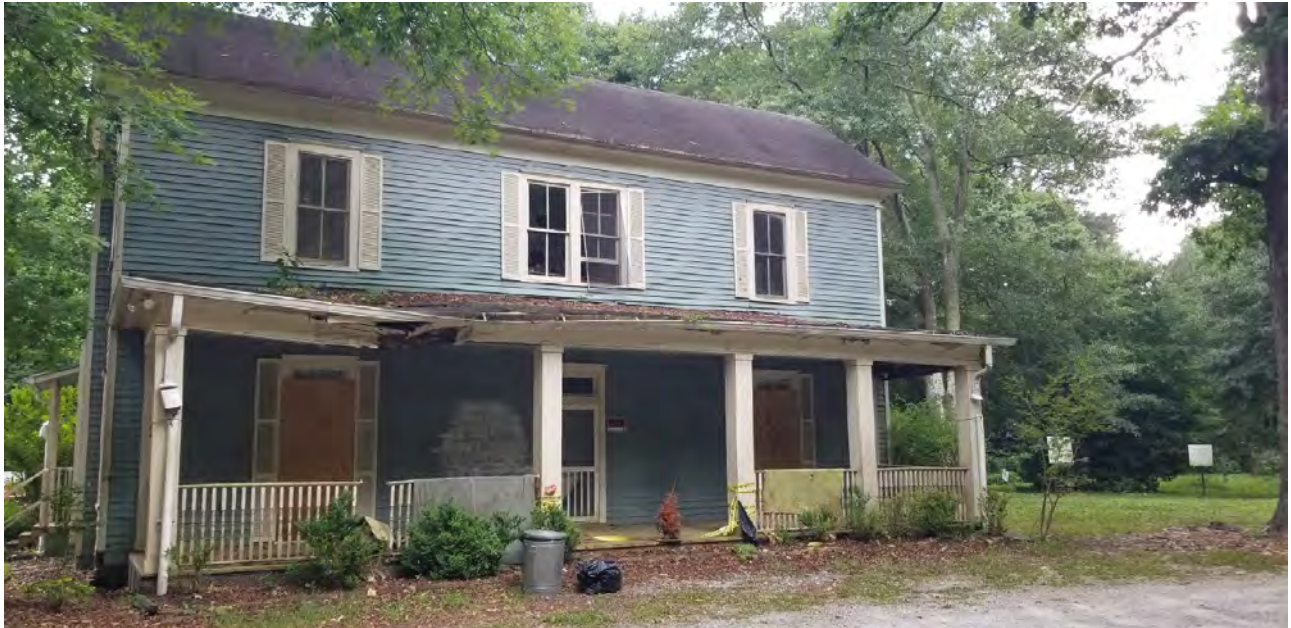
PHOTO 46: (View of North East Façade of Main Structure):
