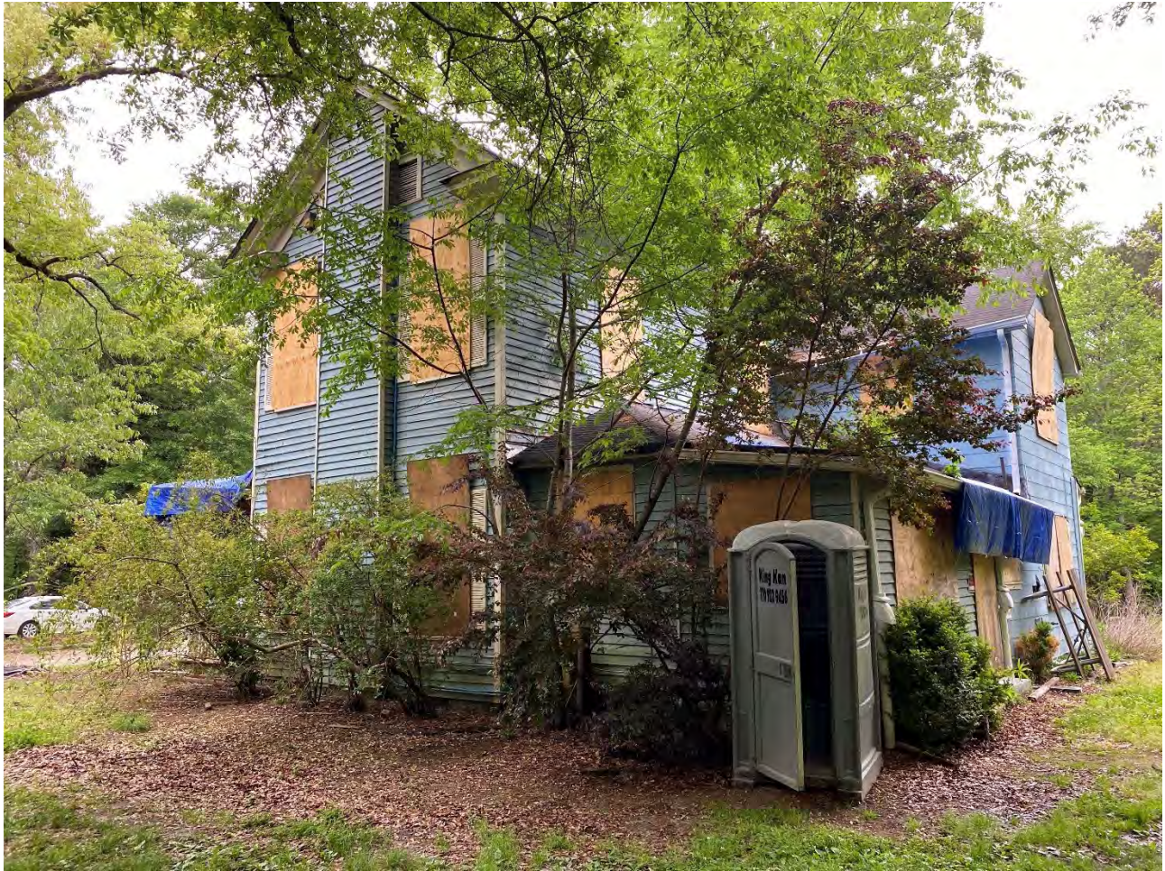
PHOTO 30: (View of Rear Corner Façade at Rear Porch): Southwest Corner.
