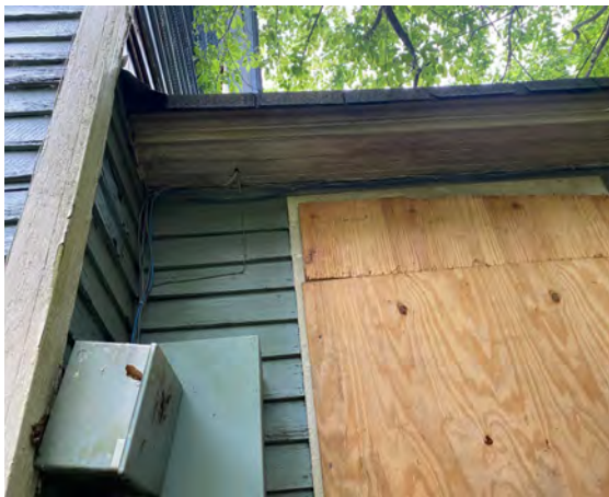
PHOTO 31, 32, & 33: (View of Rear Façade, at South West corner):
