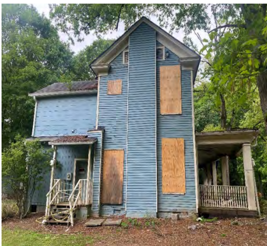
PHOTO 12: (View of East Facade):
