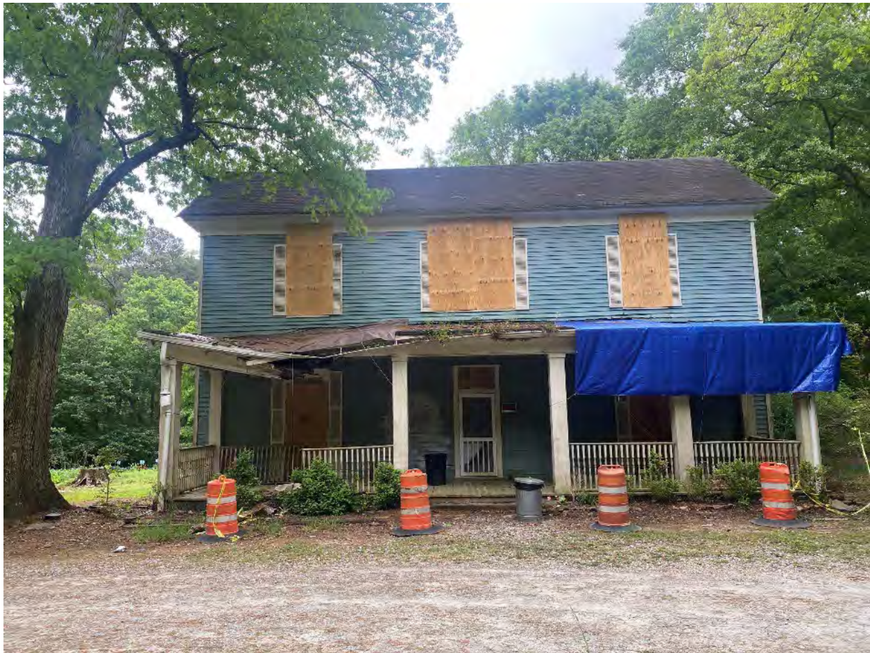
PHOTO 1: (View of North Façade, Front) - View of Building Main Structure, built in 1901.
