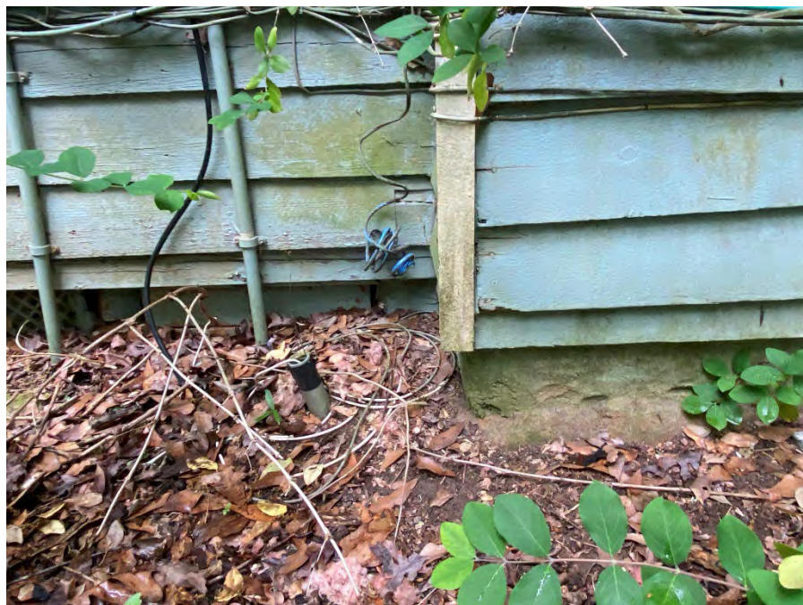
PHOTO 38 & 39: (View of West Façade at Main Structure):
