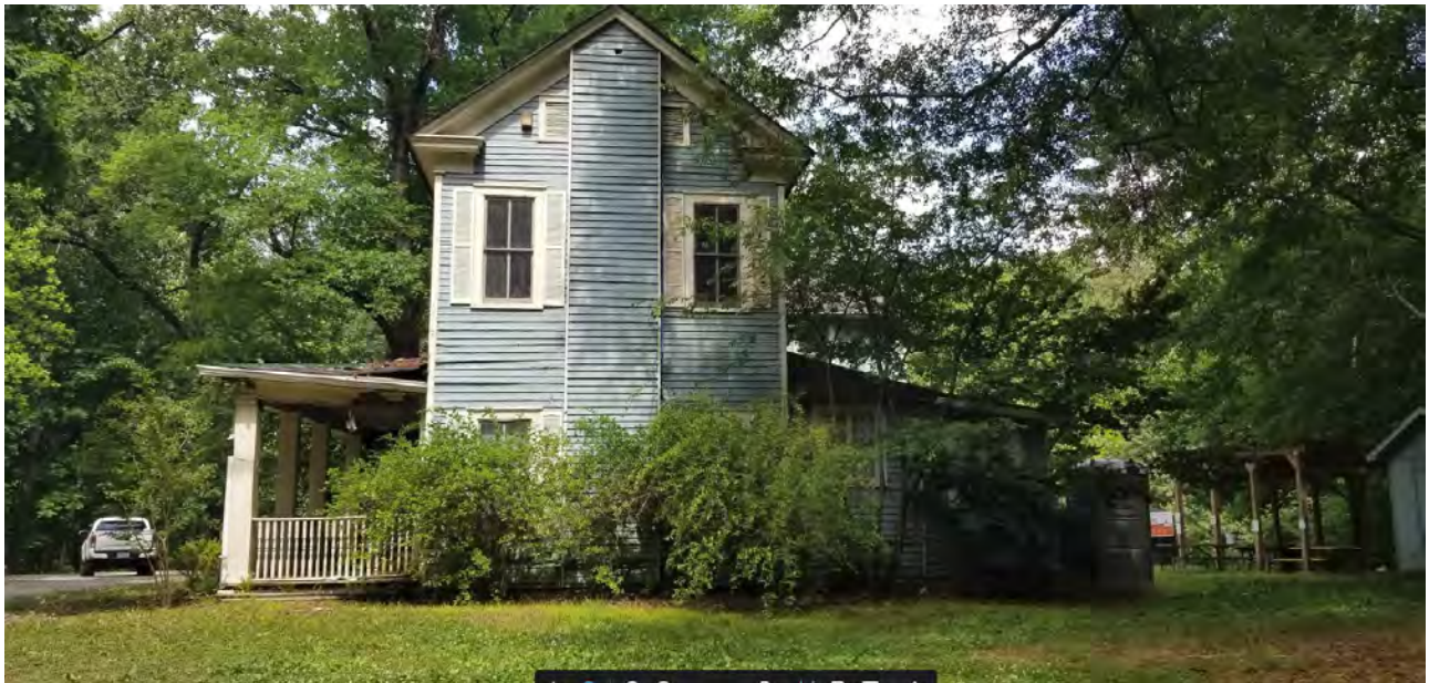
PHOTO 51: (View of West Façade at Main Structure):
