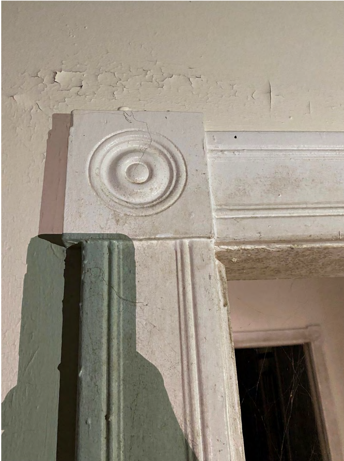
PHOTO 63: (View of Interior, Room 2, door detail):
