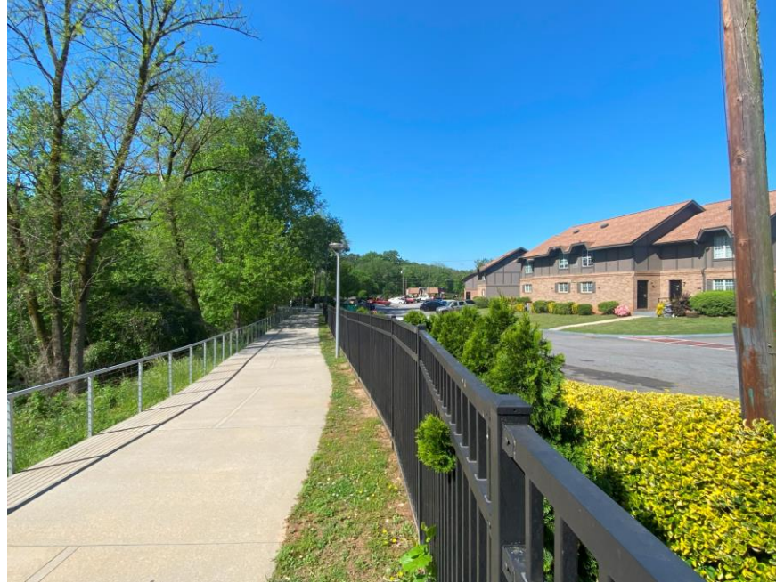
Fence along apartment easements to restrict access
