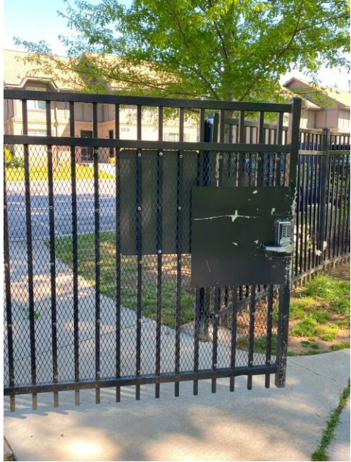
Security gate with pincode to apartments
