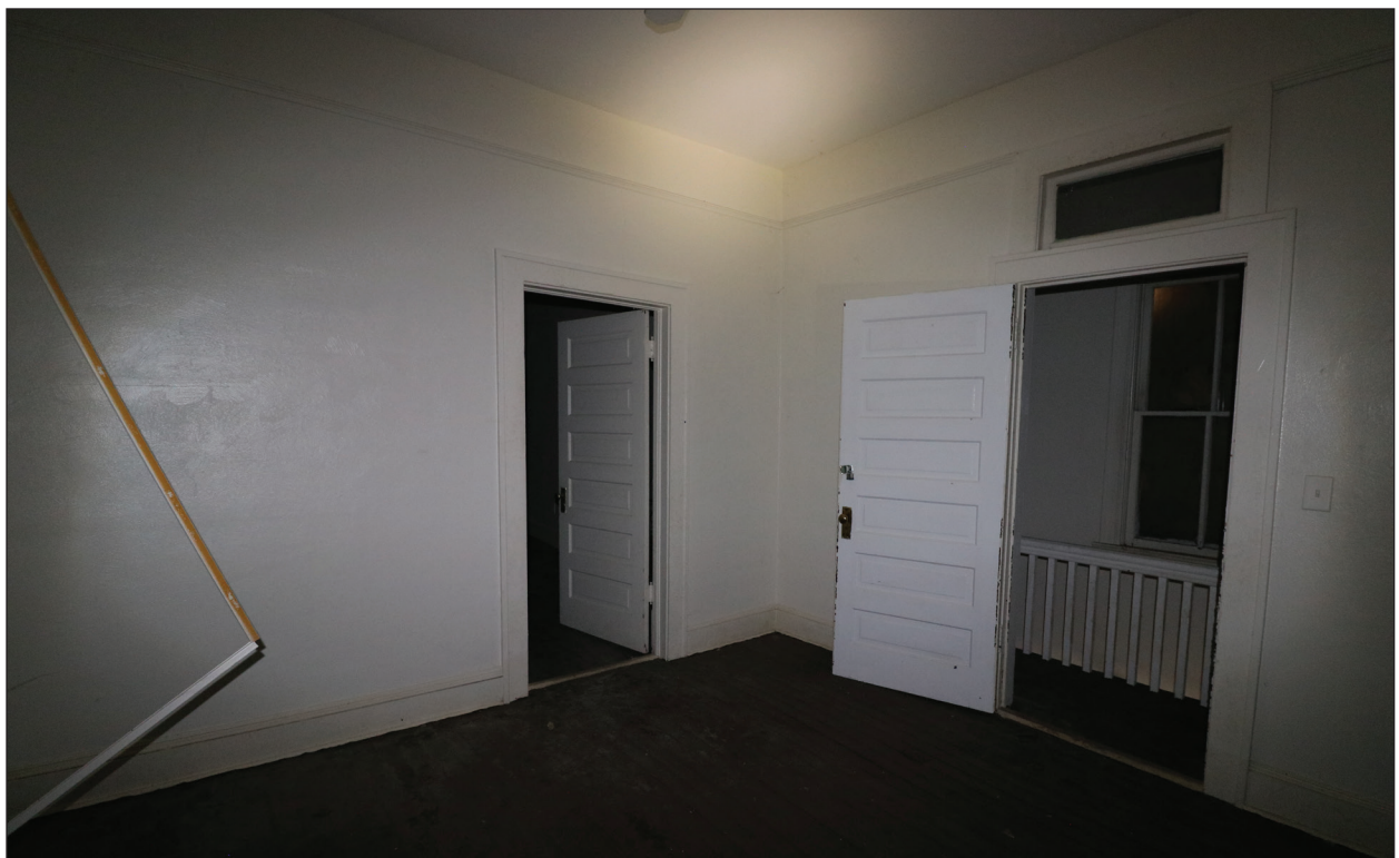
B. Second Floor Center Room, Facing Southeast
