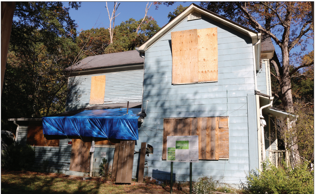
B. Rear Elevation, Facing Northwest
