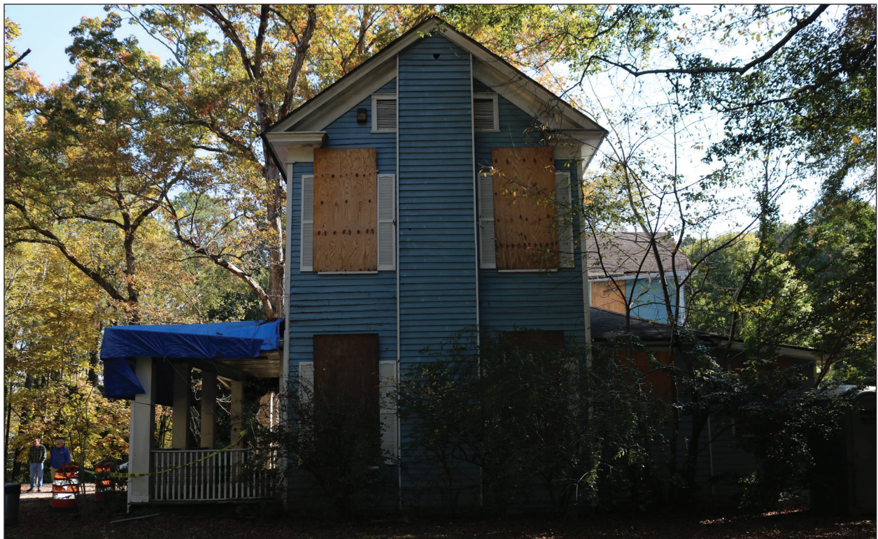
B. West Elevation, Facing East
