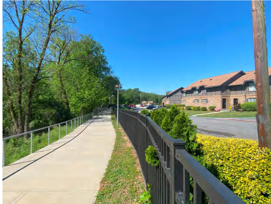
Fence along apartment easements to restrict access
