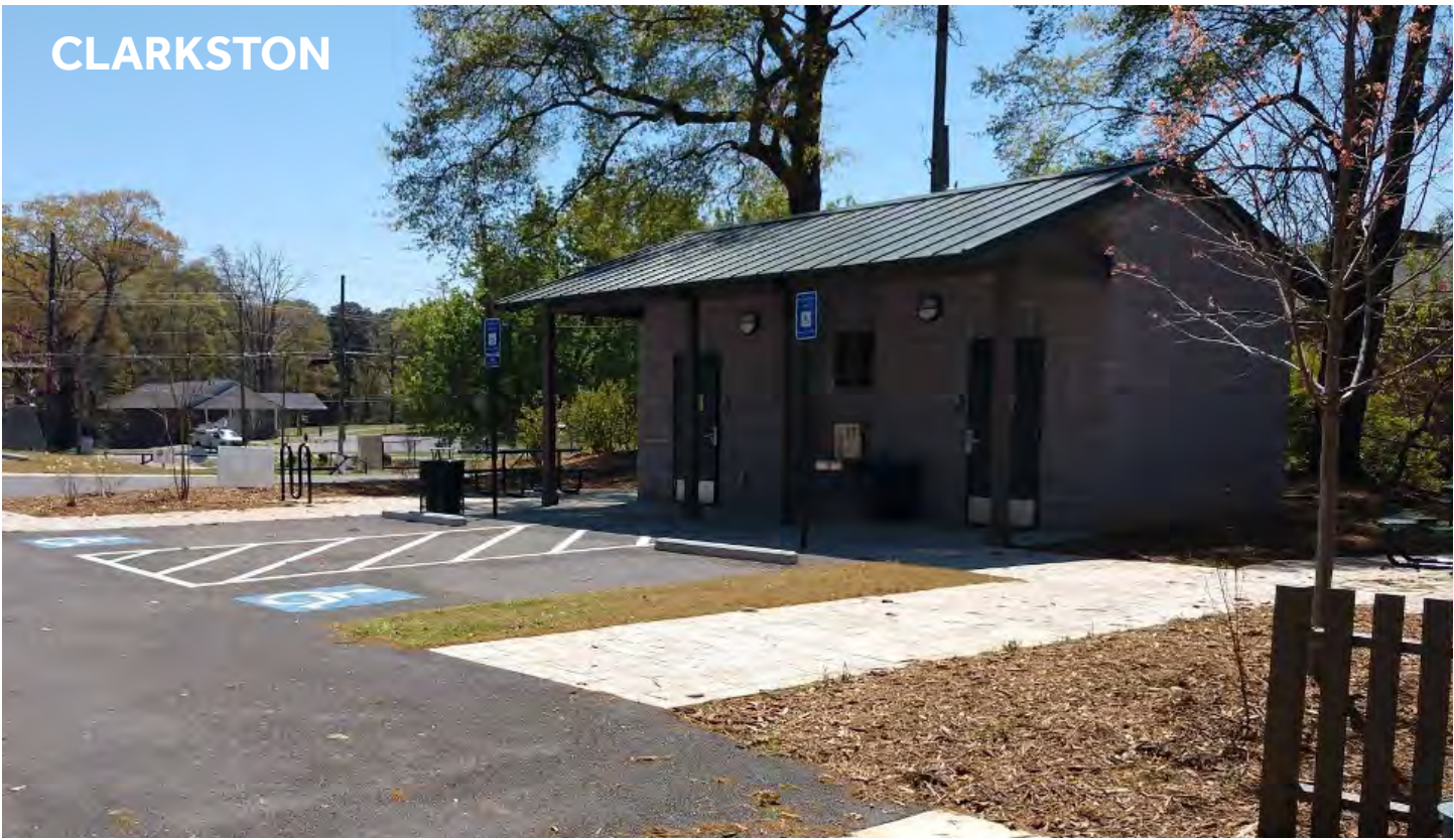
ABOVE The restroom installed at Friendship Forest in 2021 offers a high-quality standard that the City may want to establish for all future restroom projects.
